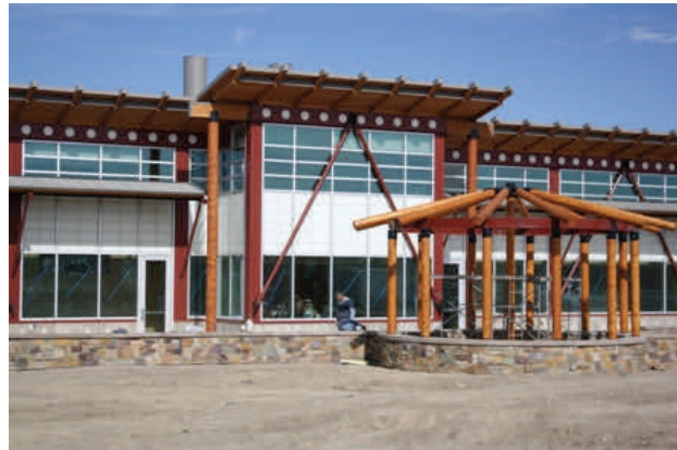
AHM-SKA-TOS-PO-II-KOH-KAN South Wind Lodge—The new math & science building on the BCC campus.
